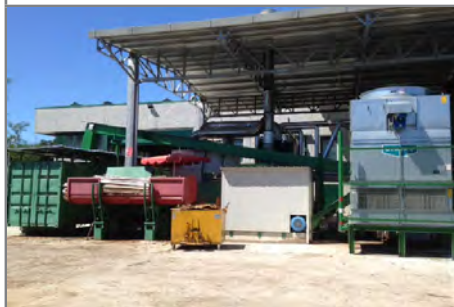
From left to right: the wood chip storage (green), the waste hopper (red),
