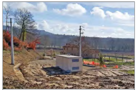
The nearby electrical cabin.
