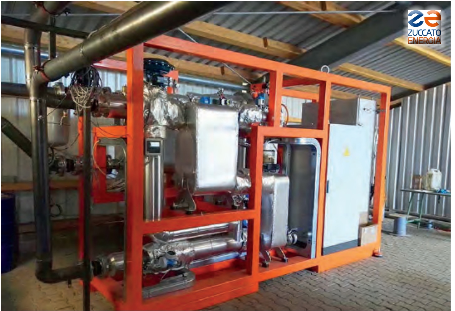
Germania 02 / Bassa Sassonia: The ORC Module seen from the hydraulic connections side
