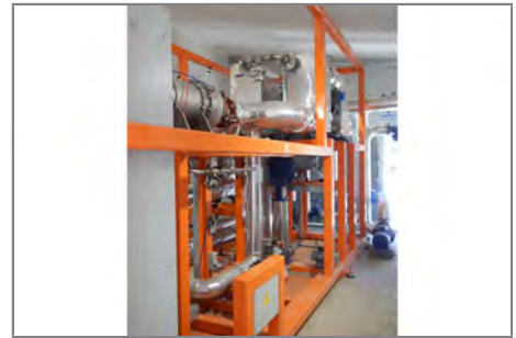
The ZE-175-LT Organic Rankine Cycle energy module, seen from the right side.
