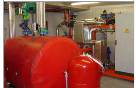
"puffer" (thermal storage tank) and the ORC module
