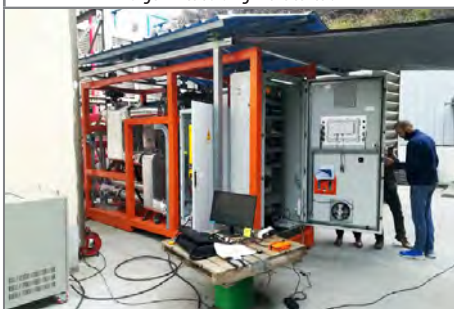
The ZE-40-ULH module during installation
