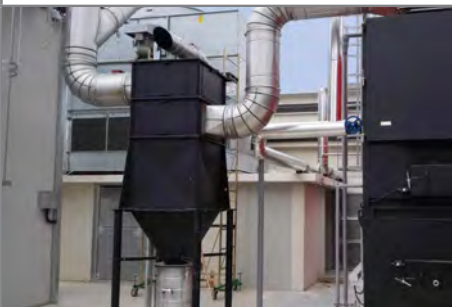
The dust trap. Wood burns cleanly, requiring only minimal flue gas treatment
