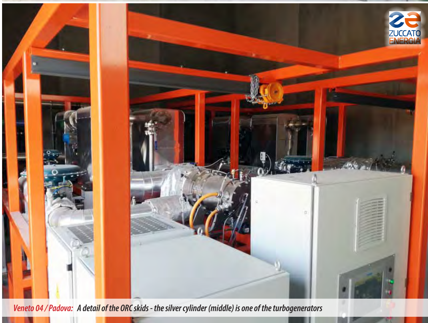
Veneto 04 / Padova: The two skid-mounted ZE-100-LT Organic Rankine Cycle modules in their room
