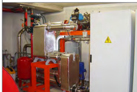
The ORC ZE-40-ULH module in greater detail
