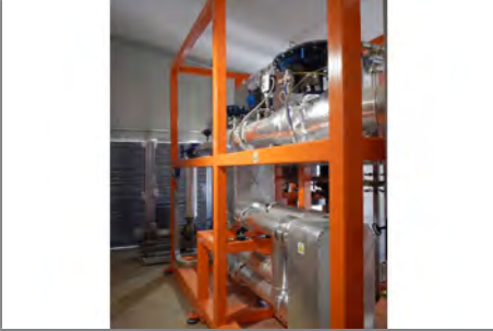
The ZE-175-LT ORC module in its skid, seen from the left side.
