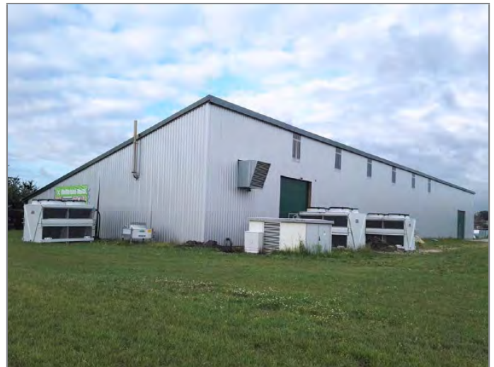
The hangar that hosts the plant
