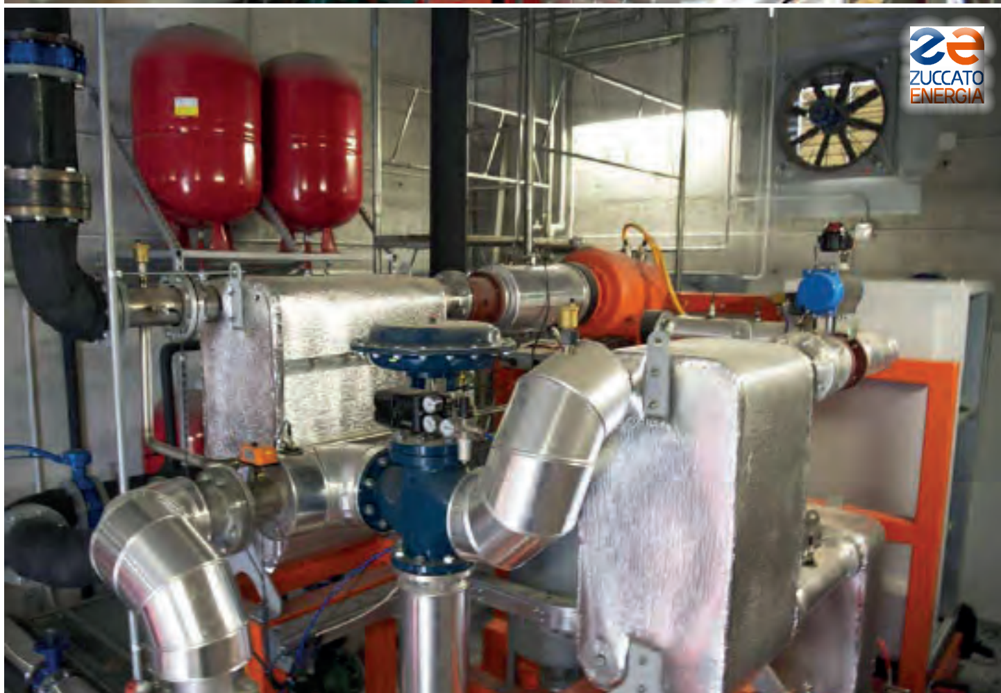
Veneto 03 / Venice: A detail of the heat exchangers of the ZE-50-ULH organic Rankine cycle module.
