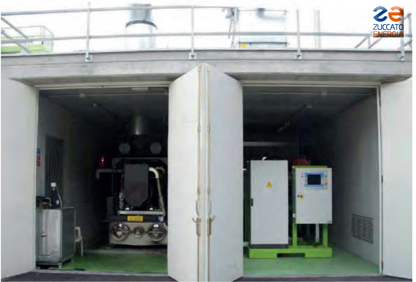
South Tyrol 01 / Bozen: The vegetable oil engine (left) and the ORC ZE-50-ULH module (right) in their concrete shelter.
