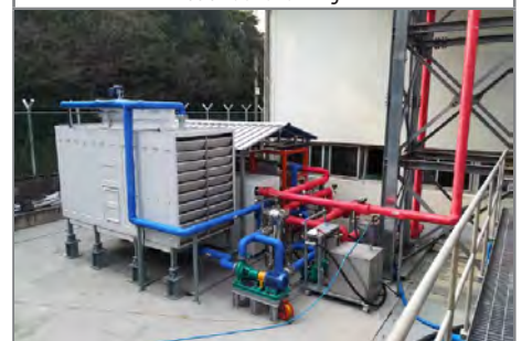
A general view of our skid installation and the cooling tower
