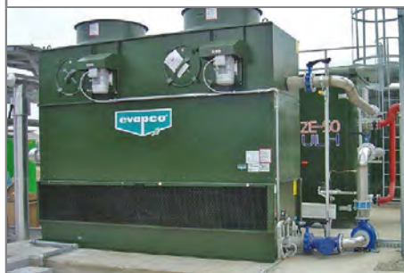
The cooling tower of the condensing stage
