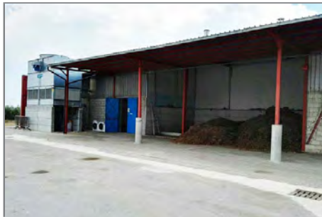
The biomass storage area
