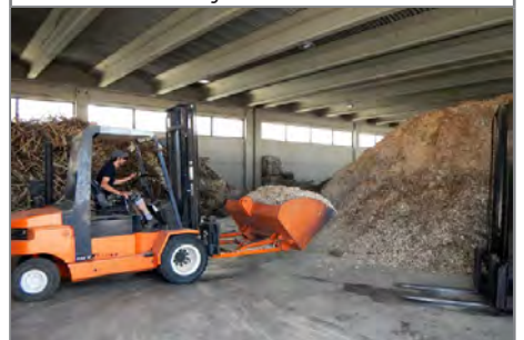
Wood chips being taken for loading in the boiler's fuel hopper.
