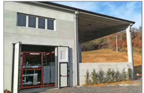
The ORC modules through the open ORC room door. The front of the power station building with the
