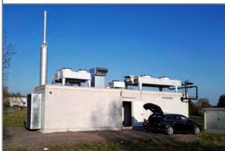
The west side of the facility with the access doorand
