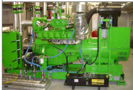
The vegetable oil engine in more detail
