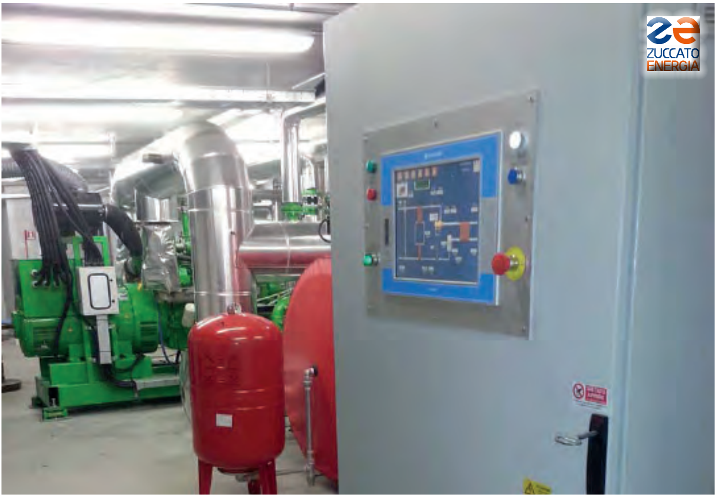
Aosta 01 / Aosta: General view of the boiler room - motor (green), thermal buffer (red) and ORC module (white)
