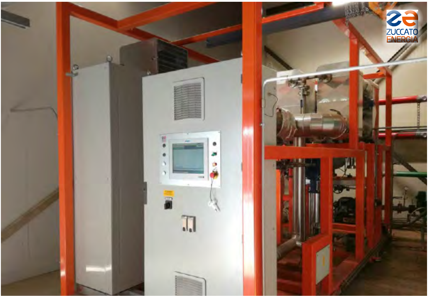
Lombardia 03 / Brescia: The ZE-150-LT organic Rankine cycle power generation module, seen from the control panel side
