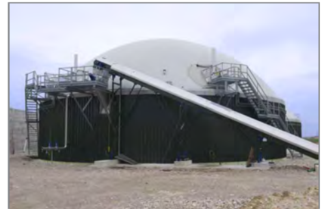
One of the two fermenters with the loading auger
