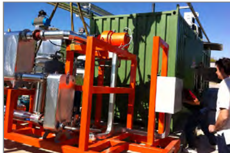
The ORC skid as it is unloaded at the site
