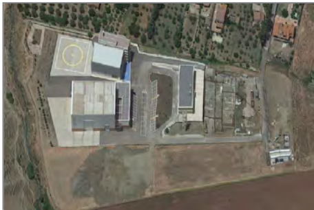
A satellite view of the faculty, with our plant in the lower right corner.
