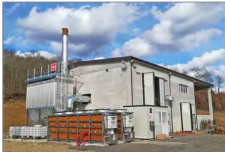
The power station building. Large door opens on boiler room, small one on ORC room.
