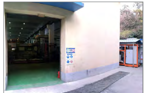
The generators building. The skid is on the right, below a small awning
