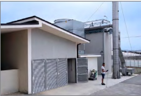
The building which hosts the ORC module. Behind, a glimpse of cooling tower and chimney.
