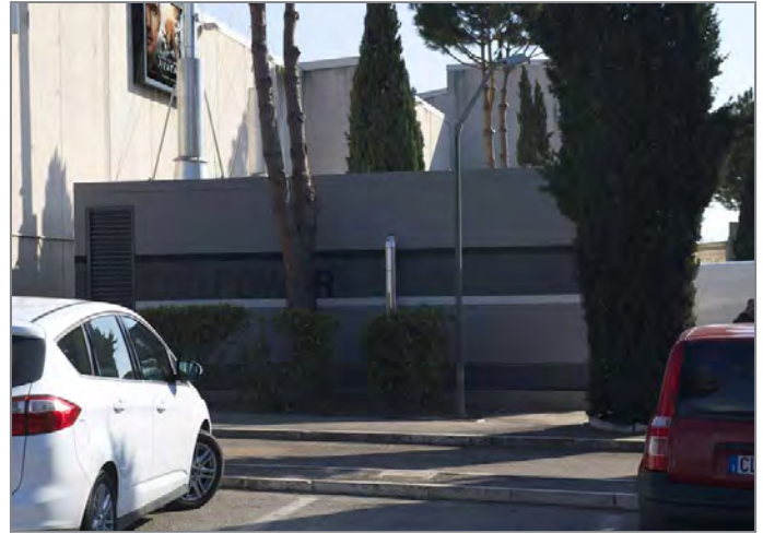
Side detail of Burkhardt cogenerators
