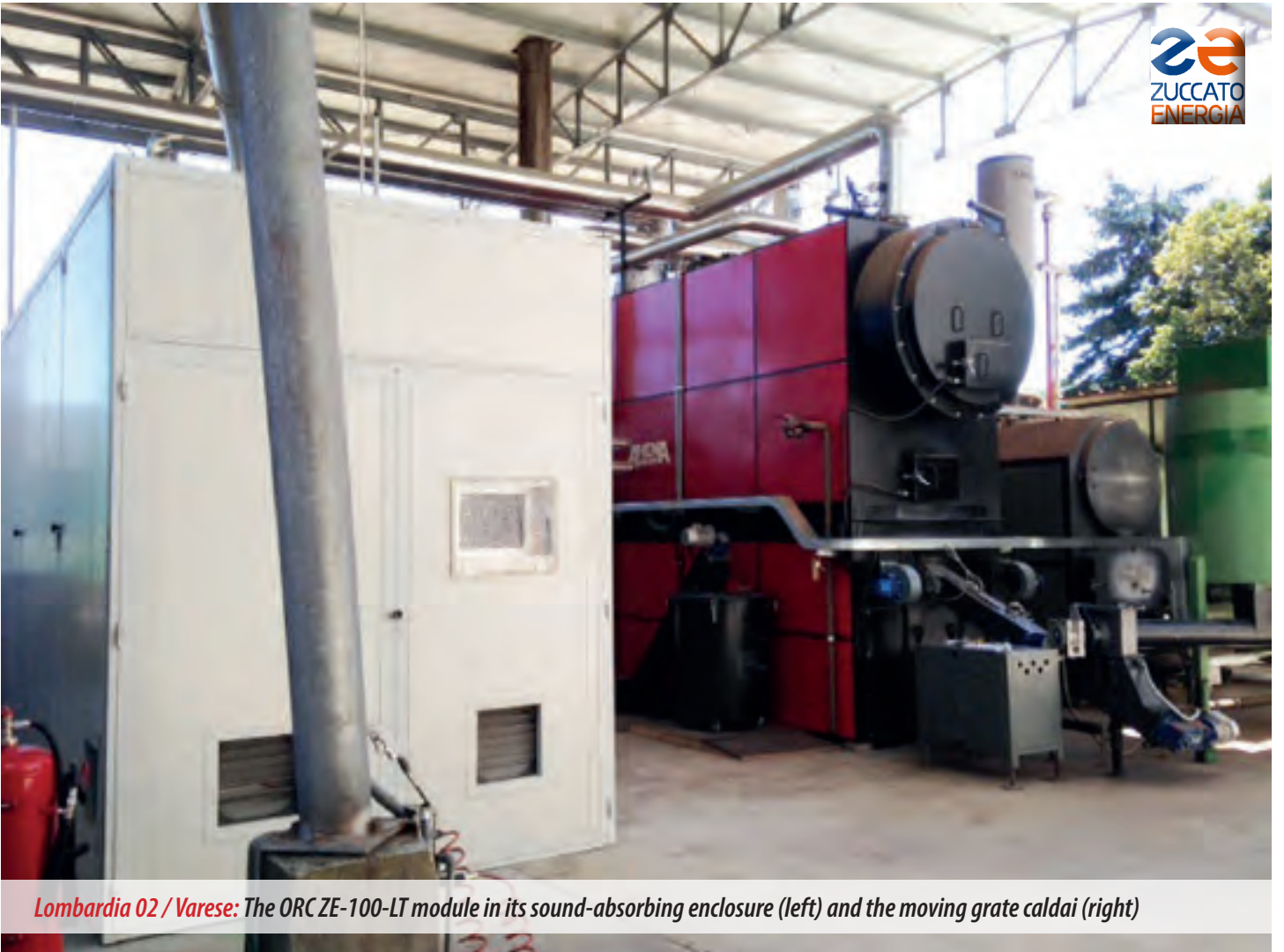
Lombardia 02 / Varese : Plant overview: ORC module (white), boiler (red) , wood chip storage and loading (green)
