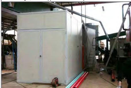
The sound-absorbing enclosure when completed.
