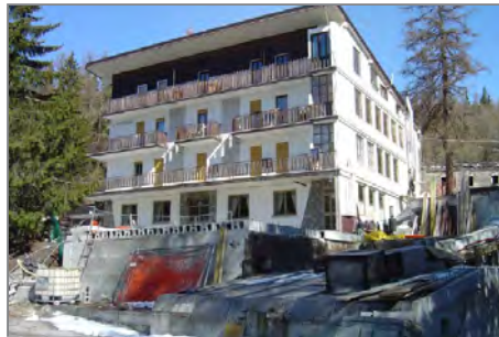
The back with the thermal power plant under construction
