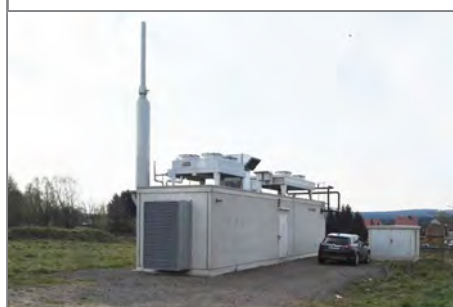
The back (south) side of the plant
