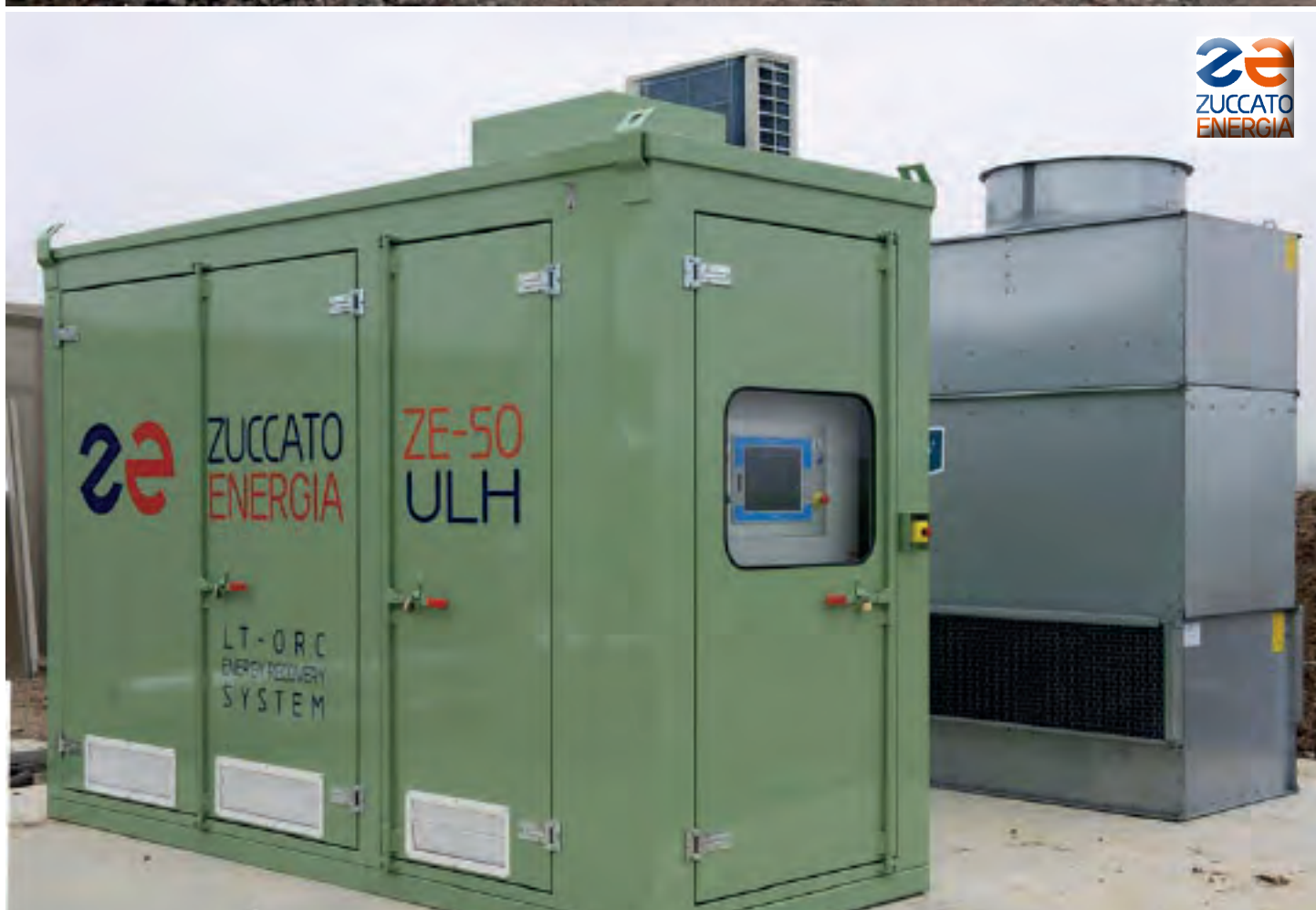
Lombardy 01 / Mantua: The weatherproof containerized ZE-50-ULH module; in the background, the cooling tower.
