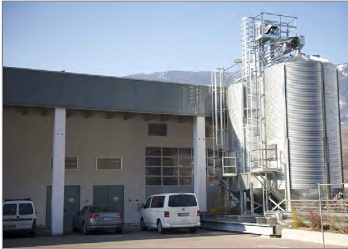
General aerial view of the complex
