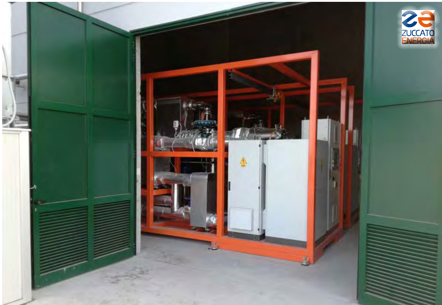
Veneto 04 / Padova: The two skid-mounted ZE-100-LT Organic Rankine Cycle modules in their room
