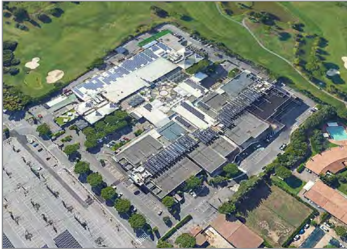
General aerial view of the complex
