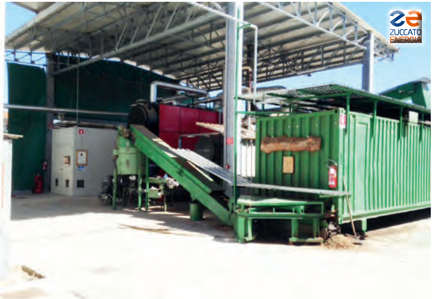
Lombardia 02 / Varese : Plant overview: ORC module (white), boiler (red) , wood chip storage and loading (green)
