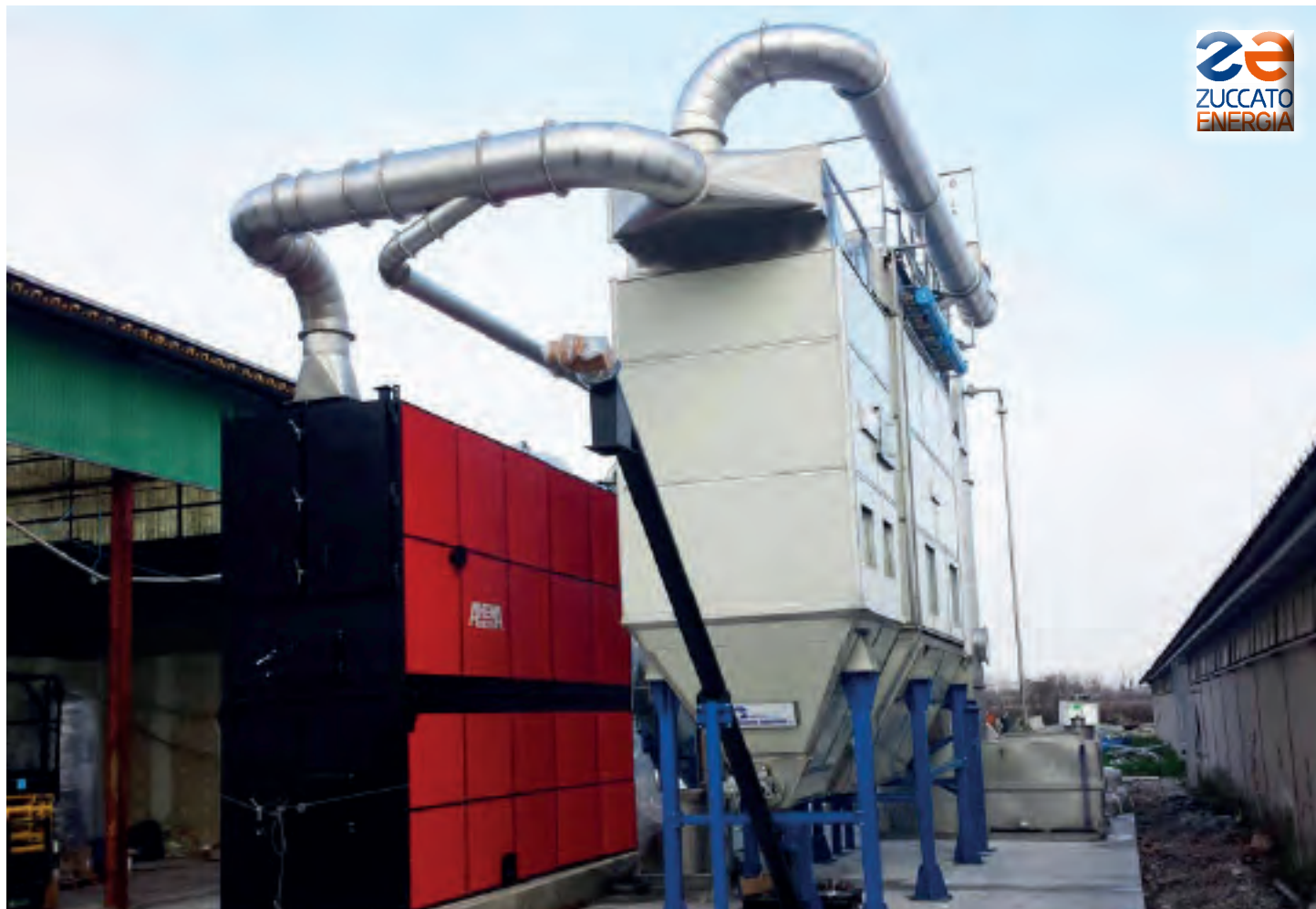
Friuli 01 / Pordenone: The Manure-fired moving grate boiler(left) and the flue gas treatment system.
