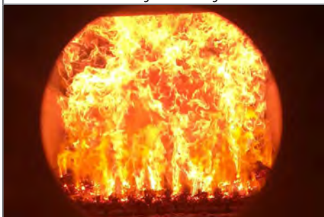
A peek inside the operating boiler.
