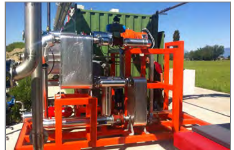
Side view of the plant
