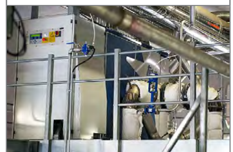
Detail of one of Turbec's hot air turbines
