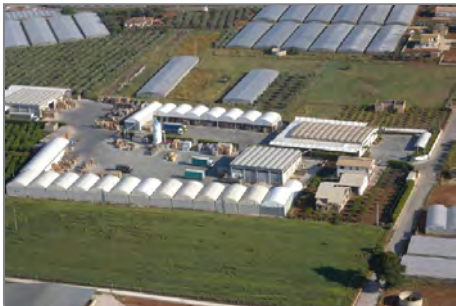
An aerial overview of the site.
