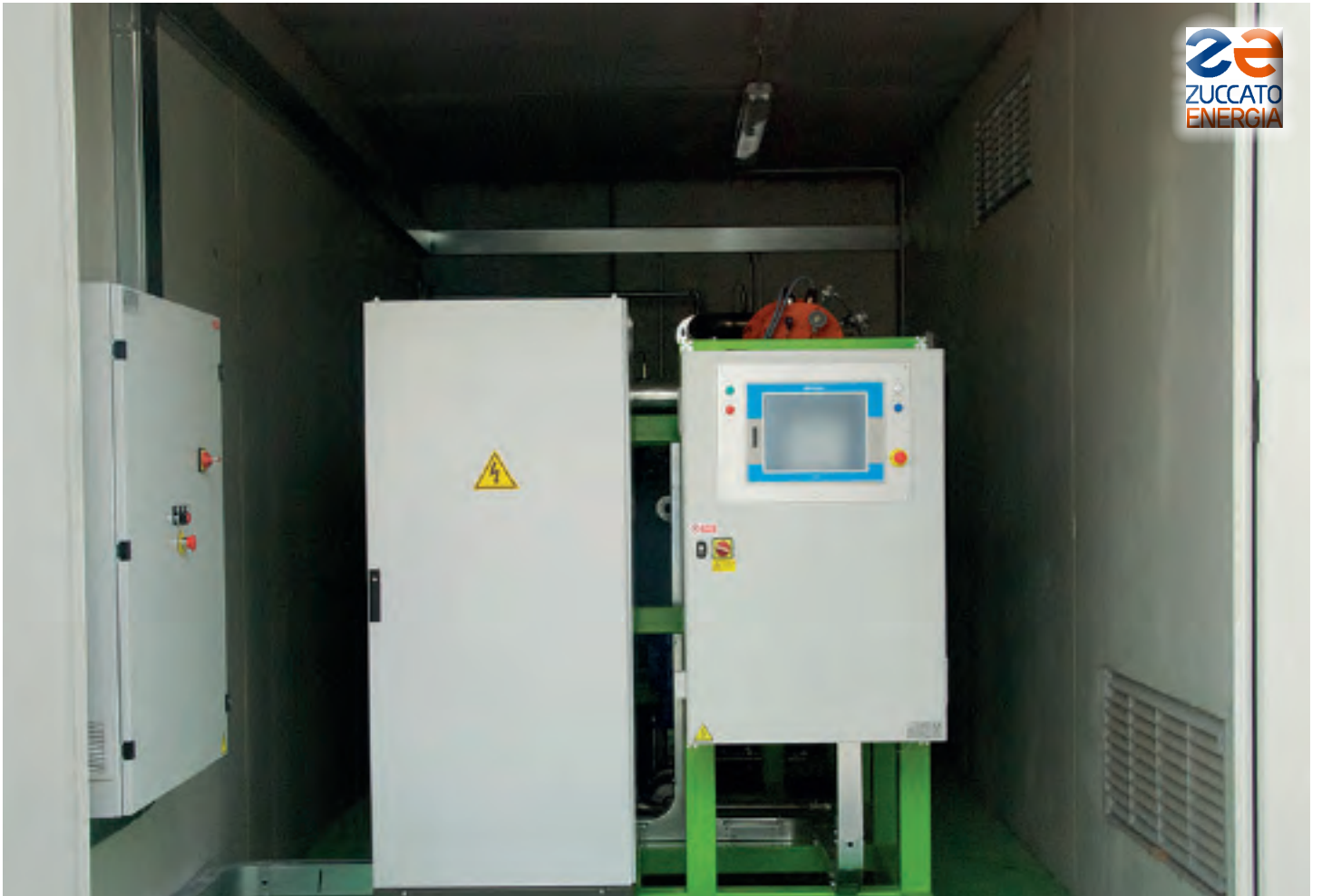
South Tyrol 01 / Bozen: A detail of the ZE-50-ULH organic Rankine cycle module in its room.
