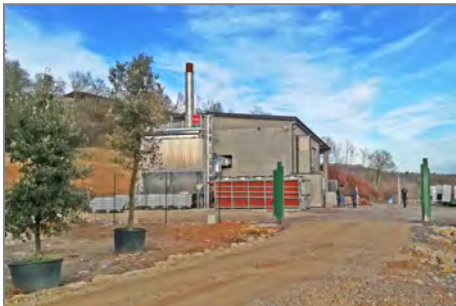
The power station entrance gate.
