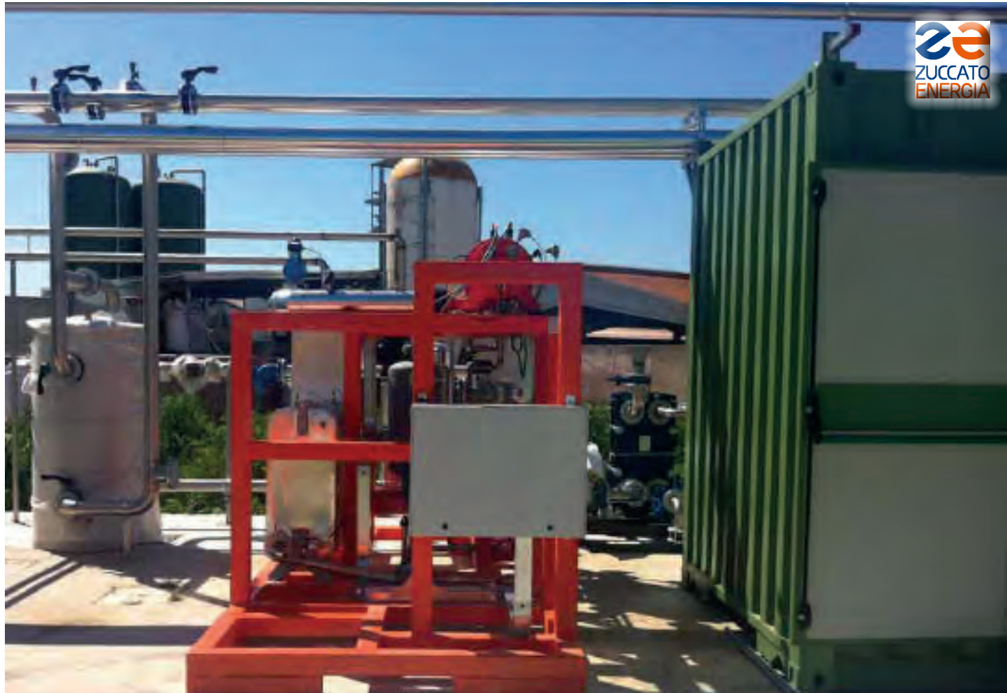
Veneto 02 / Padoua: The ORC ZE-50-ULH module seen from the front.
