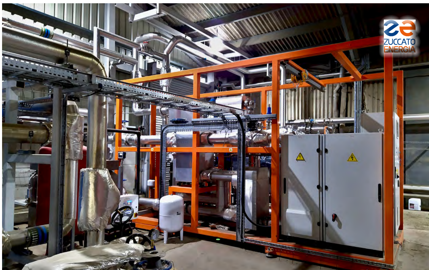
United Kingdom 01 : The ZE-105-CHP module in place
