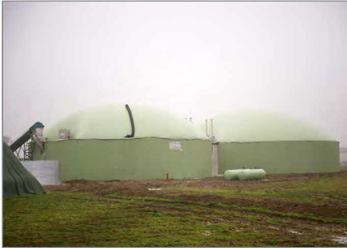
General view of fermentation tanks
