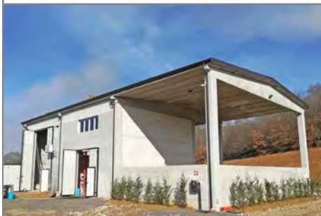
The front of the power station building with the biomass storage area in foreground.
