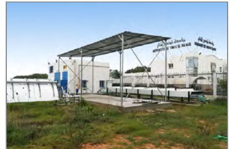
The white building protecting the skid (L).
