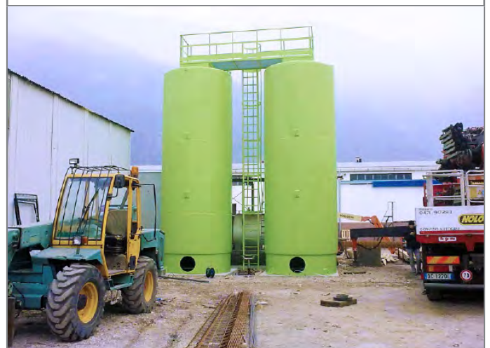
Vegetable oil tanks during installation.
