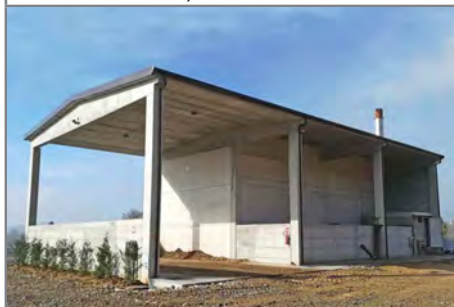
The rear of the power station with (L to R) biomass storage, fuel hopper and control room door.
