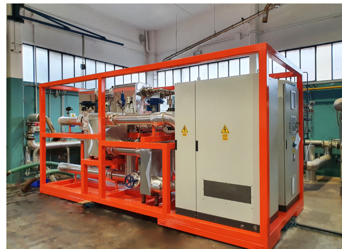
ORC System - Test Area for final testing
